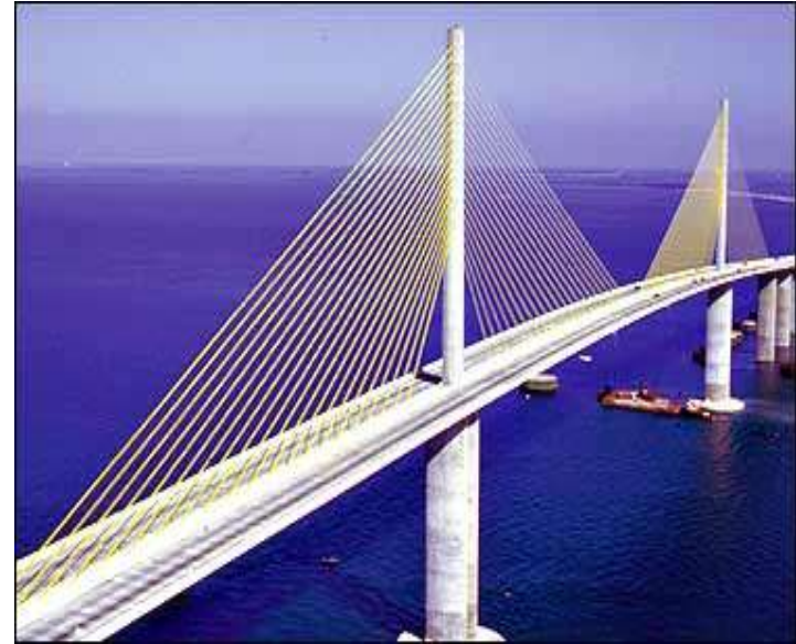
Foto: Sunshineskyway Bridge, Florida
